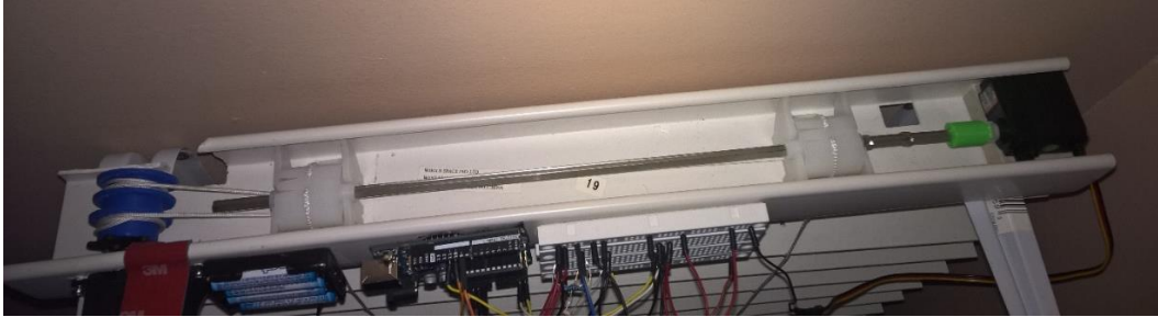
The head-rail after all modifications – Fig. 10
